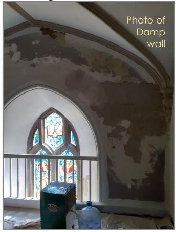
Right: Photo of High level (clear storey) window which is newly painted. A plastic strip has been fitted at the base of the window to prevent condensation draining down on to the paintwork of the wall. The weep hole to allow the condensation to drain outside has been restored. A further problem has arisen in that the electrical cables along the base of the south and north walls, which supply power, are faulty and will have to be replaced. These extras will add to the cost of the project.
