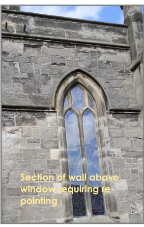
poor condition and the opportunity will be taken to rake out the joints and repoint usina lime mortar which will enable the wall to dry out fully over time.
